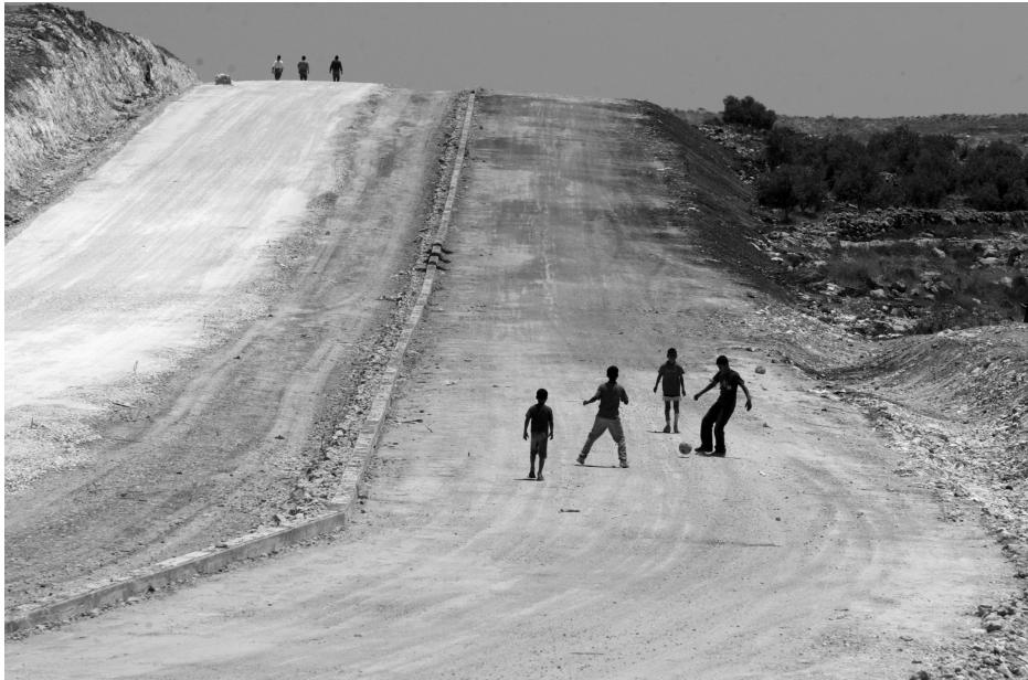
Palestinian boys play soccer at the construction site of Israel's separation wall near the West Bank village of Biddu, 30 June 2004. (Ammar Award/Reuters)
